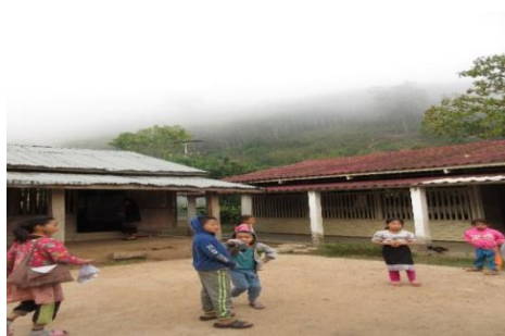
Photo 7. A primary school in Village L
